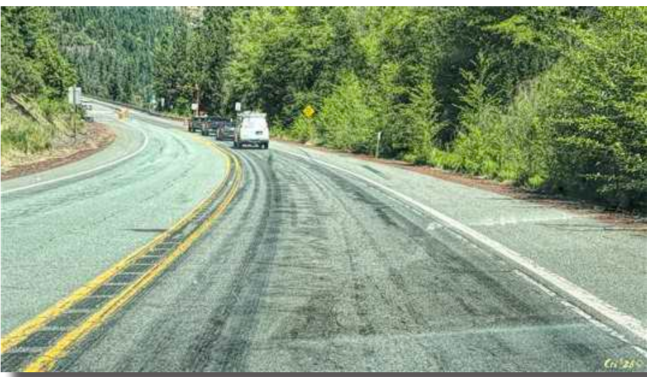
Clearly a lot of drivers have made very sudden stops - mostly staying in the lane at least - mostly - as they approach the temporary stop light installed for the constuction on the bridge over Lost Creek Lake.
